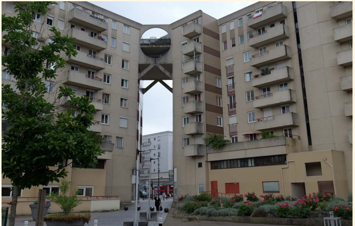
Figure 3.4: Large scale housing scheme at St Quentin-en-Yvelines new town south east of Paris. Source: Photograph by Susan Parham, 2025
