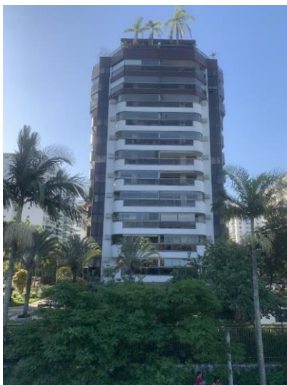
Figure 6.5 New residential developments adjacent to Rio's Olympic Park. (Source: Author)
