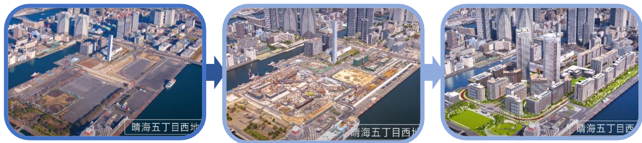
Figure 4.2 Overview of the Tokyo 2020 Olympic and Paralympic Village, highlighting the transformation from an international trade centre to the athletes' village to Harumi Flag Residential development (Source: Tokyo Metropolitan Government).
