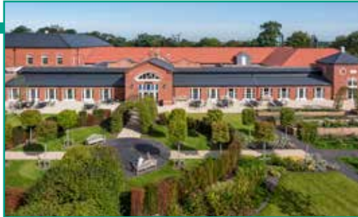
Defence and National Rehabilitation Centre submitted by Arup and BS Stanford Ltd A state of the art clinical rehabilitation facility providing injured service men and women with a place to recover and rebuild their lives. Image by Andreas von Einsiedel Archive Ltd.
