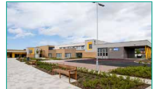
The Jean Bishop Integrated Care Centre submitted by Hull City Council A transformative hub delivering integrated care to older people and emergency services, co-located within the heart of the community alongside specialist housing via multi-agency partnership. Image by Citycare Ltd.
