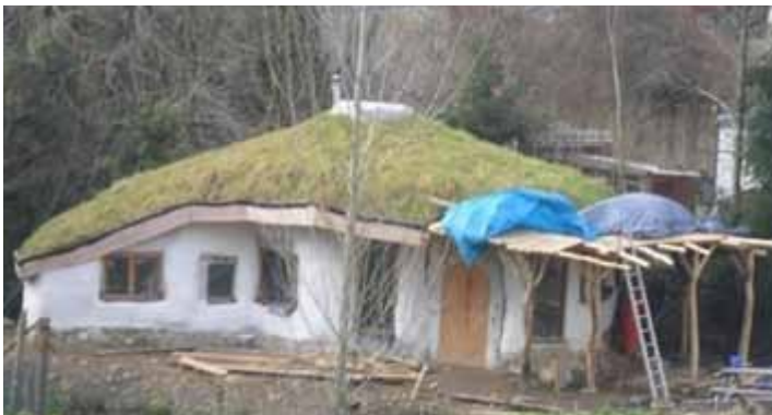
Above: Pwll Broga under construction in 2012 at Trecwnc, Glandwr Pembrokeshire, which received planning permission on appeal in 2015, after initially being investigated as an unauthorised development in the countryside.
