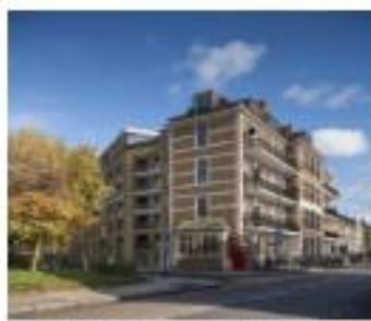
QUEEN ELIZABETH HOSPITAL TOWER HAMLETS, LONDON
