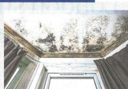
Tenants are trapped in squalid housing in this Weston-super-Mare block. One of them, Jade*, is seen amid black mould and peeling wallpaper. Photographs by Stephen Shepherd/the Observer
