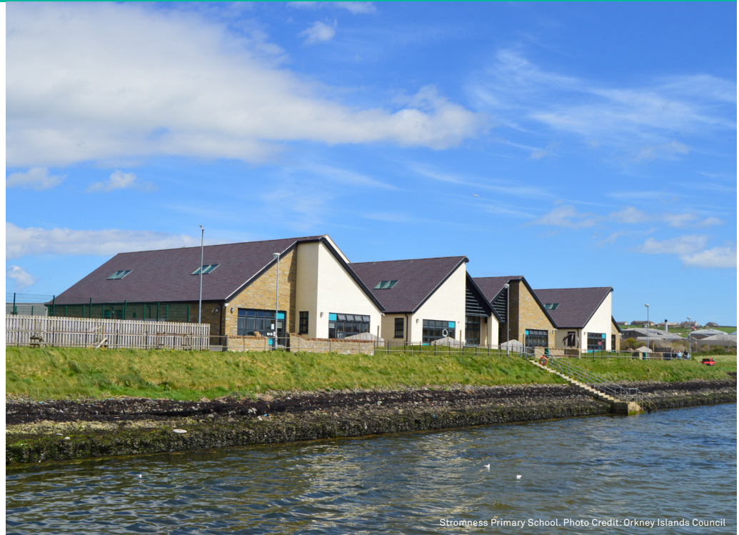
Stromness Primary School. Photo Credit: Orkney Islands Council
