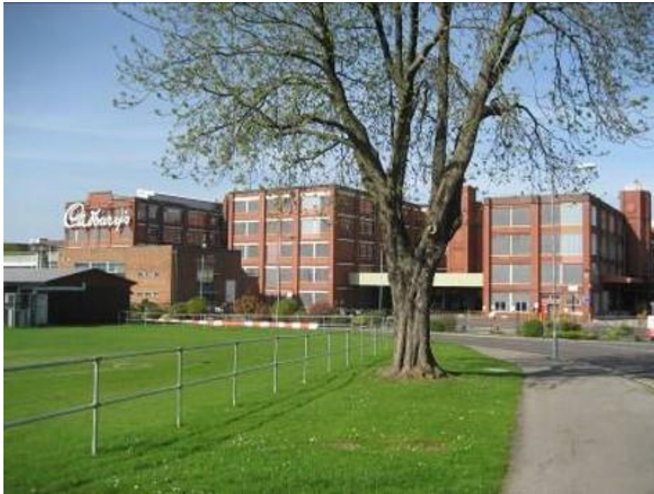
Previous development – factory buildings
