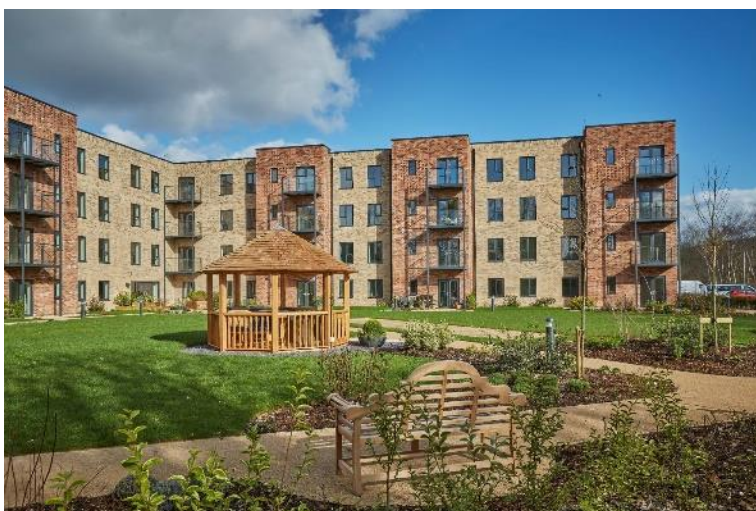
External view of Jacobs Gate. Image credit: Gladman Retirement Living
