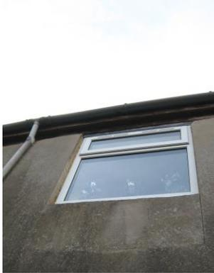
1. Remove the upvc window shown in the photograph and replace with single glazed, side hung casement with one horizontal glazing bar of 20mm per casement. The glazing shall be secured with putty.
