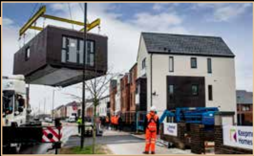
ilke Homes ilke Homes are one of the UK's largest volumetric modular house builders at the forefront of delivering sustainable and beautiful homes using MMC.
