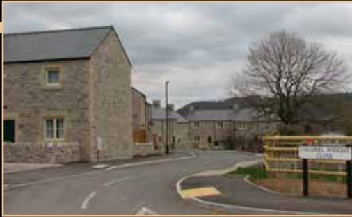
Colonel Wright Close, Bakewell submitted by Peak District National Park Authority Colonel Wright Close is a high quality development of 30 affordable local needs houses on an important gateway site in the Peak District National Park.
