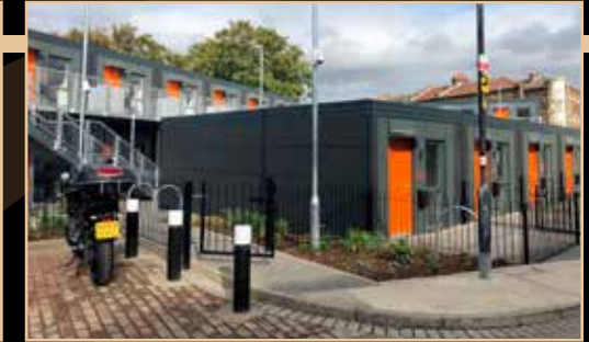
Olive Morris Court, Homeless Accommodation submitted by Sphere25 A modular unit development to support 32 homeless people within Haringey, with on-site support and management, and 16 homes being gifted to the Council.
