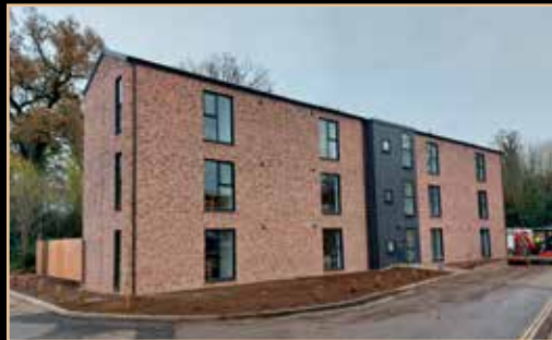
Webster Court submitted by Bidwells Webster Court provided rapid development of affordable housing to address homelessness in Norwich through dynamic partnership working with the local authority and developer. Image by Broadland Housing Association.
