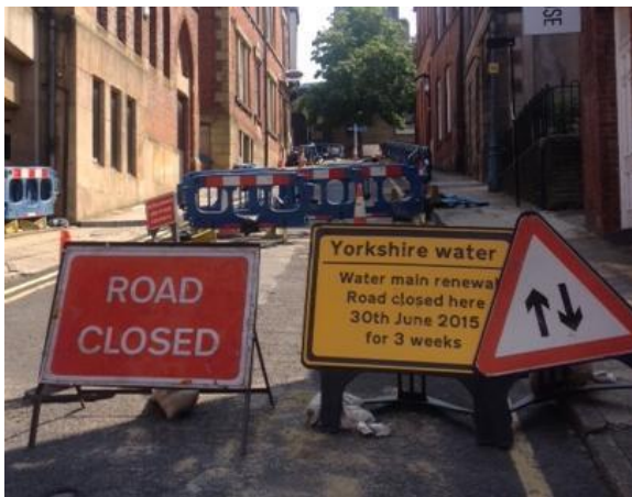
Sewers and public utilities
