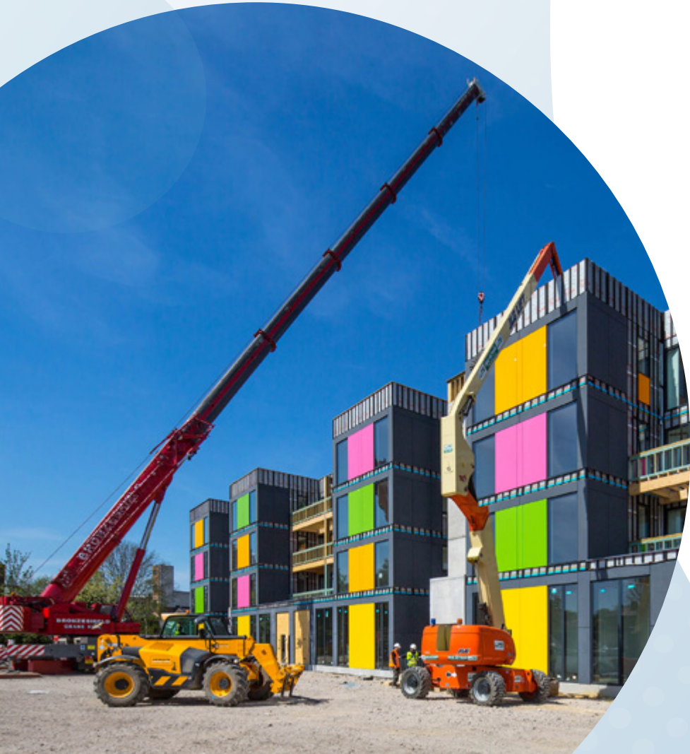
Place Ladywell construction. Credit: Rogers Stirk Harbour Partners
