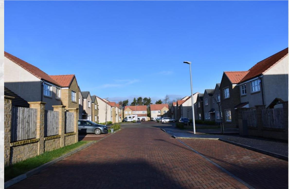
Streetscape Gateside West, Haddington
