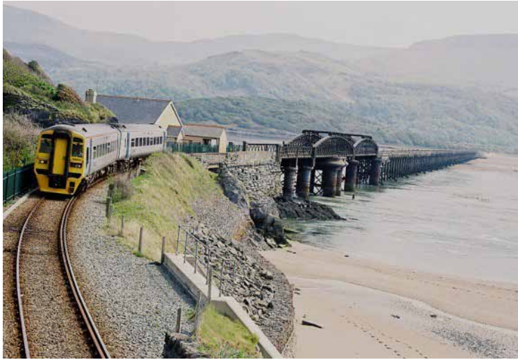
Above: Rail Bridge across the Maddawch Estuary
