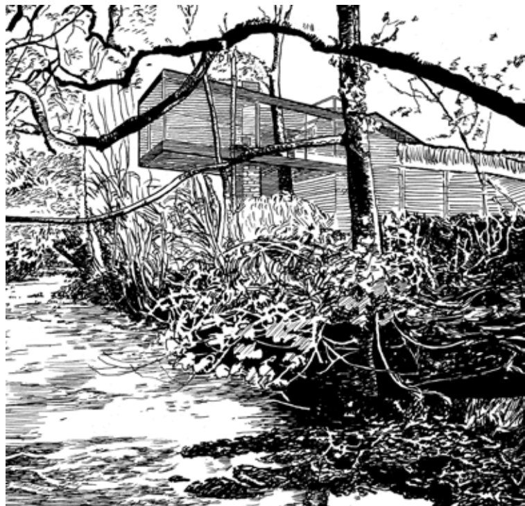
Above: The main living space in this house in Brecon is cantilevered towards the river. The timber and steel frame structure is clad with Welsh slate and local timber. Resource-saving features include high thermal mass, grass roofs, solar panels, wood-chip boiler and recycled grey water. Drawing by Rob Cowan.
