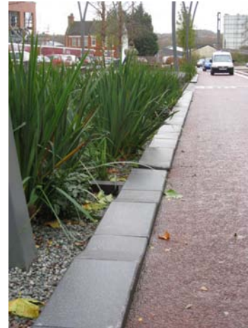
West Street - SUDS
