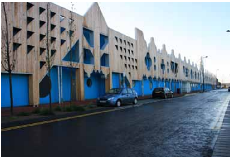
Above: Part of the Porth Teigr area in Cardiff Bay
