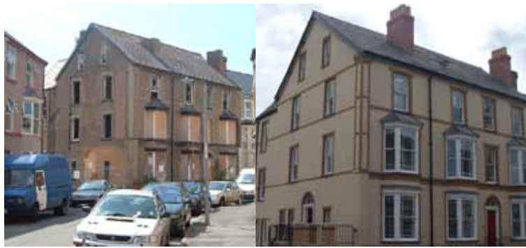
Above: Before and after of 16-18 Edward Henry Street, Rhyl
