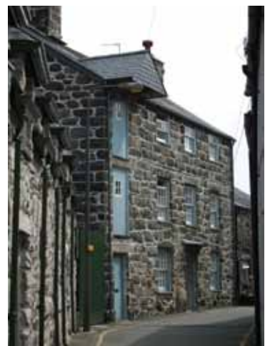
Above: Cambrian Mill is one of the many buildings that reflect Dolgellau's importance as a textile-producing centre © Cadw, Welsh Government (Crown Copyright)
