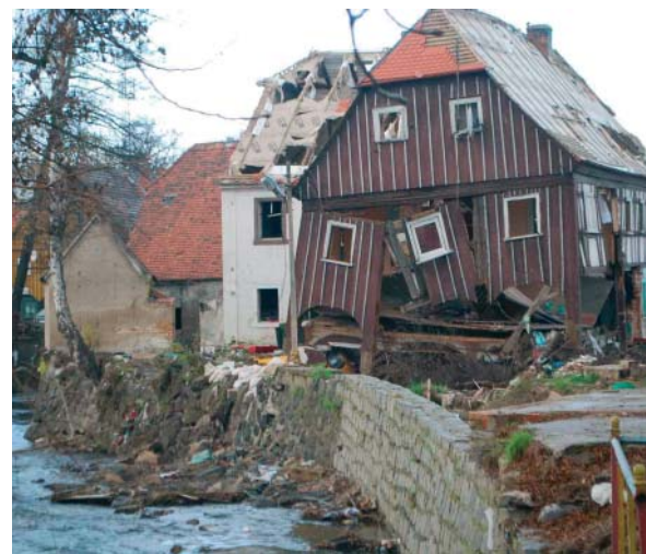
Flood damage at Bogatynia.
