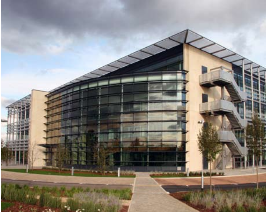
The Hub: solar shading and water heaters raised headquarters sustainability rating
