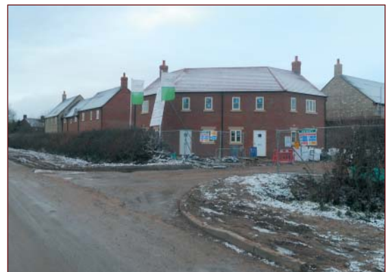
Harbury scheme after; nearing completion.
